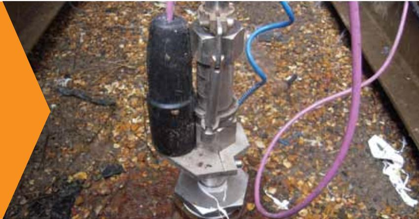
Hydroguard<sup>®</sup> is a well-established and proven 24 hour monitoring and protection system for water trunk mains. The cost effective, battery operated system continuously measures and transmits flow, pressure and noise data by SMS or GPRS, providing fast notification of any unusual activity or suspected bursts.
